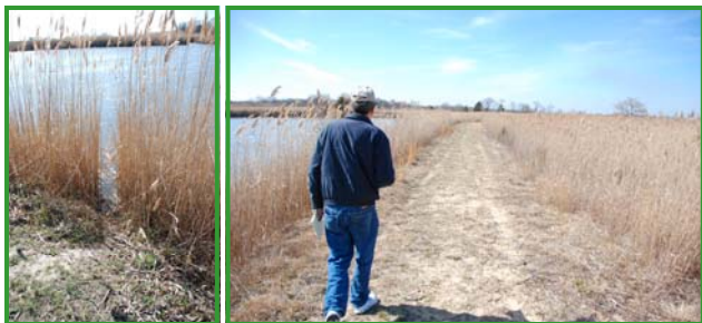
Locust Island Meadow Bank Company Levee at Hancock's Bridge
